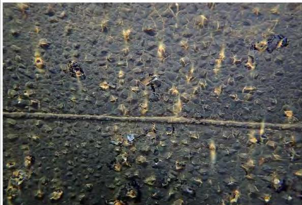
**Conclusion/Discrepancies:** Coating is severely blistered, most of which have cracked open and corrosion is forming. Sandblast and recoat in the immediate future
