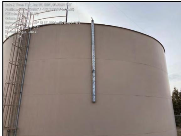
**Photograph 3.4 Juniper Tank (Tank 1) showing manual tank level gauge.**
