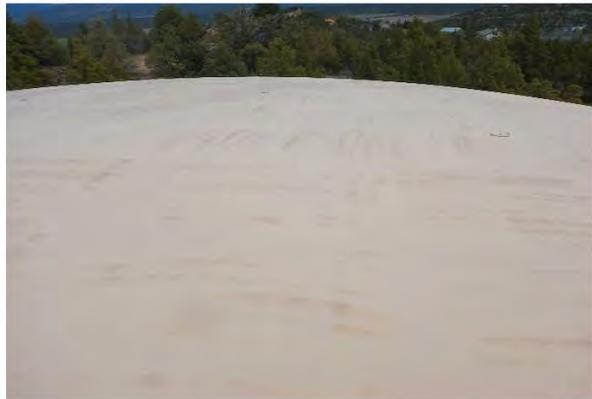
Conclusion/Discrepancies: The coating is oxidized and thin, the primer is exposed with indications of corrosion starting to form.
