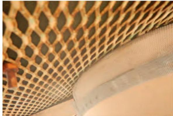
Conclusion/Discrepancies Screen in place and well secured Vent is in good condition no problematic concerns
