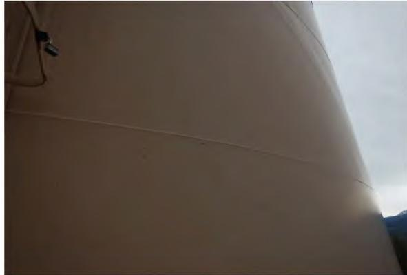
Conclusion/Discrepancies Minor nicks and scratches, no coating adhesion problems shell is in satisfactory condition
