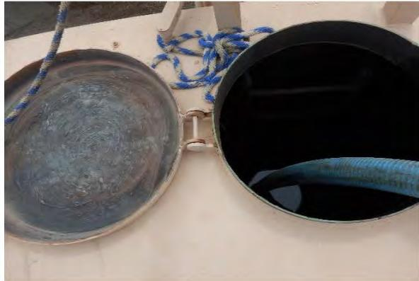
Conclusion/Discrepancies Needs a gasket put in place, minor corrosion where gasket should be
