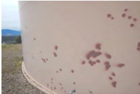
**Conclusion/Discrepancies** Nicks and scratches that need touch up. Many areas already corrected and appears to be holding up with no corrosion present
