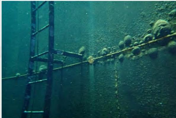
**Conclusion/Discrepancies:** Weld seams are heavily blistered with corrosion present above the water line corrosion and cracking more extensive
