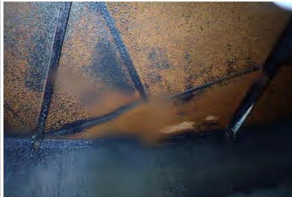
**Conclusion/Discrepancies:** Surface corrosion covers the plates as well as the trusses and hardware. Coating has failed and needs to be sandblasted and recoated
