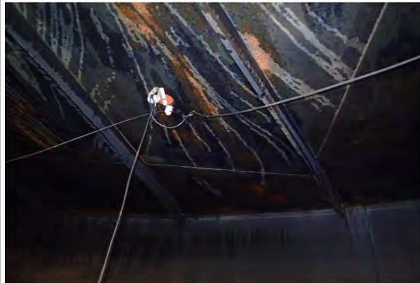
**Conclusion/Discrepancies:** Surface corrosion covers the plates, minor corrosion on the trusses and hardware. Coating is at the end of its service life and needs redone
