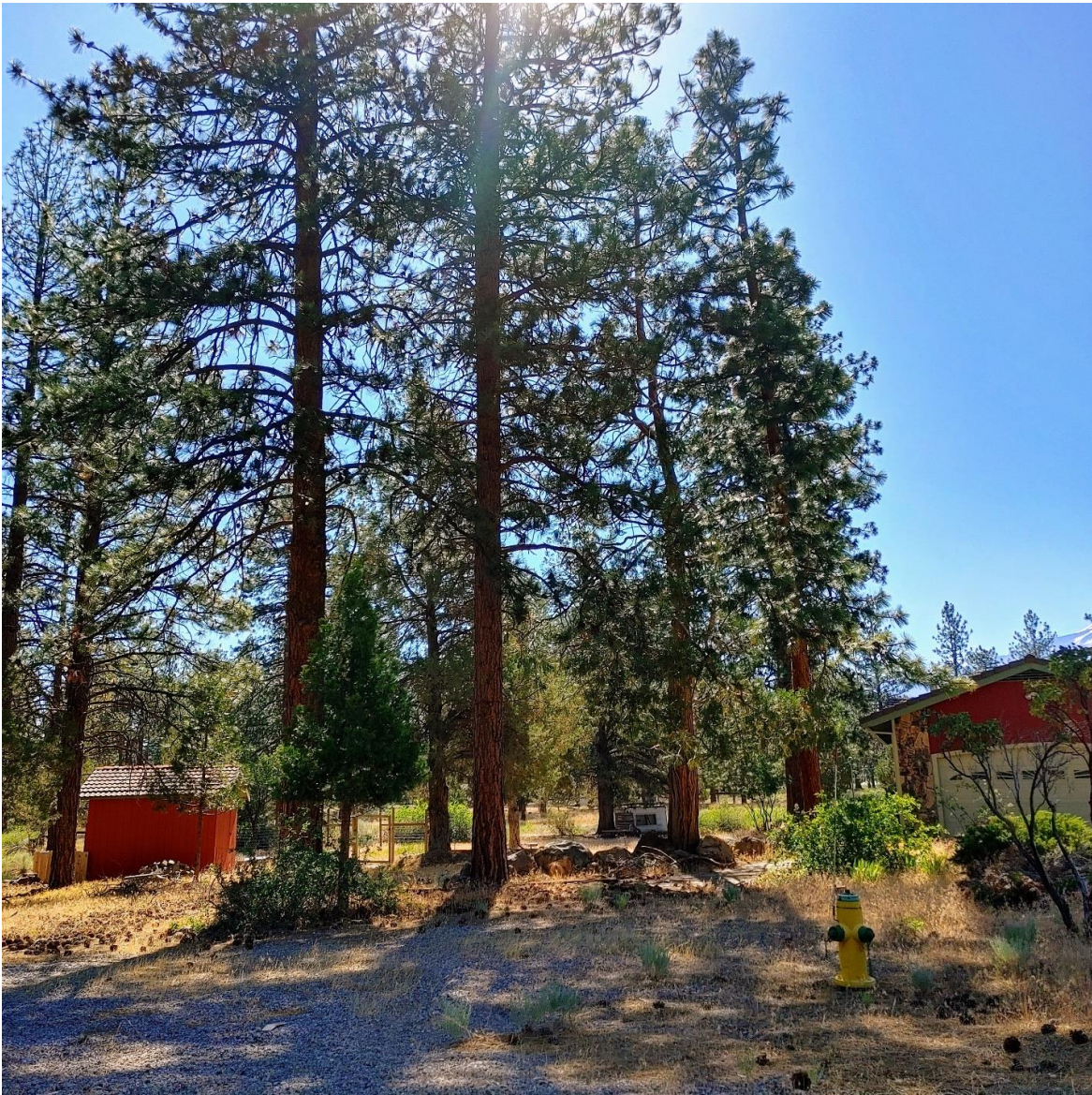
Photo 8: Looking east from Jack Rabbit Road onto fire hydrant #175 that will be replaced with a new fire hydrant. This fire hydrant is surrounded by small rabbit brush, gravelly soil, and ponderosa pine. The soil directly around the fire hydrant will be disturbed as all parts of the hydrant will be replaced down to the elbow in the ground.
