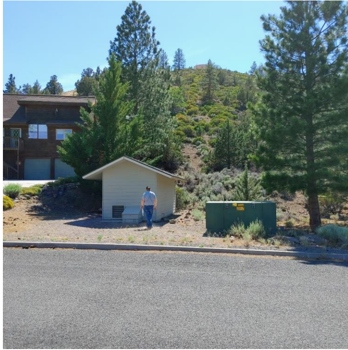
Photo 1: Looking west at pump station 53 on Palmer Drive where the location of the temporary water tank outside of the building would be placed as water tank 4 is upgraded to a bigger size. Water tank #4 can be seen on top of the slope. Gravel is observed on the east side of the pump station where the temporary water tank would be placed. Photo taken: 6/22/2022.
