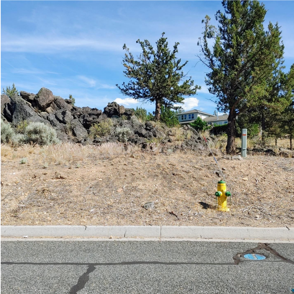
Photo 7: Looking east from Mountain Wood Drive onto fire hydrant #275 that will be replaced with a new fire hydrant. This fire hydrant is surrounded by asphalt, large rocks, gravelly soil, and juniper trees. The soil directly around the fire hydrant will be disturbed as all parts of the hydrant will be replaced down to the elbow in the ground.
