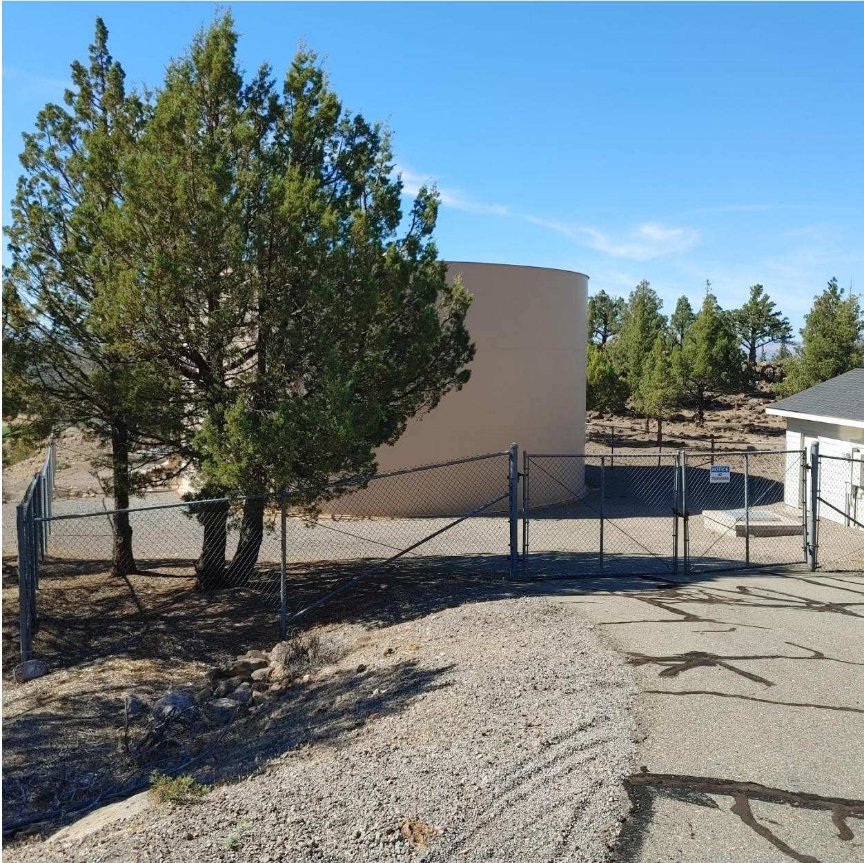
Photo 3: Looking north west from Stone Crest Drive at water tank #3 which is surrounded by small rocks, gravel, and juniper trees. Water tank #3 will be re-painted. Photo taken: 6/22/2022.
