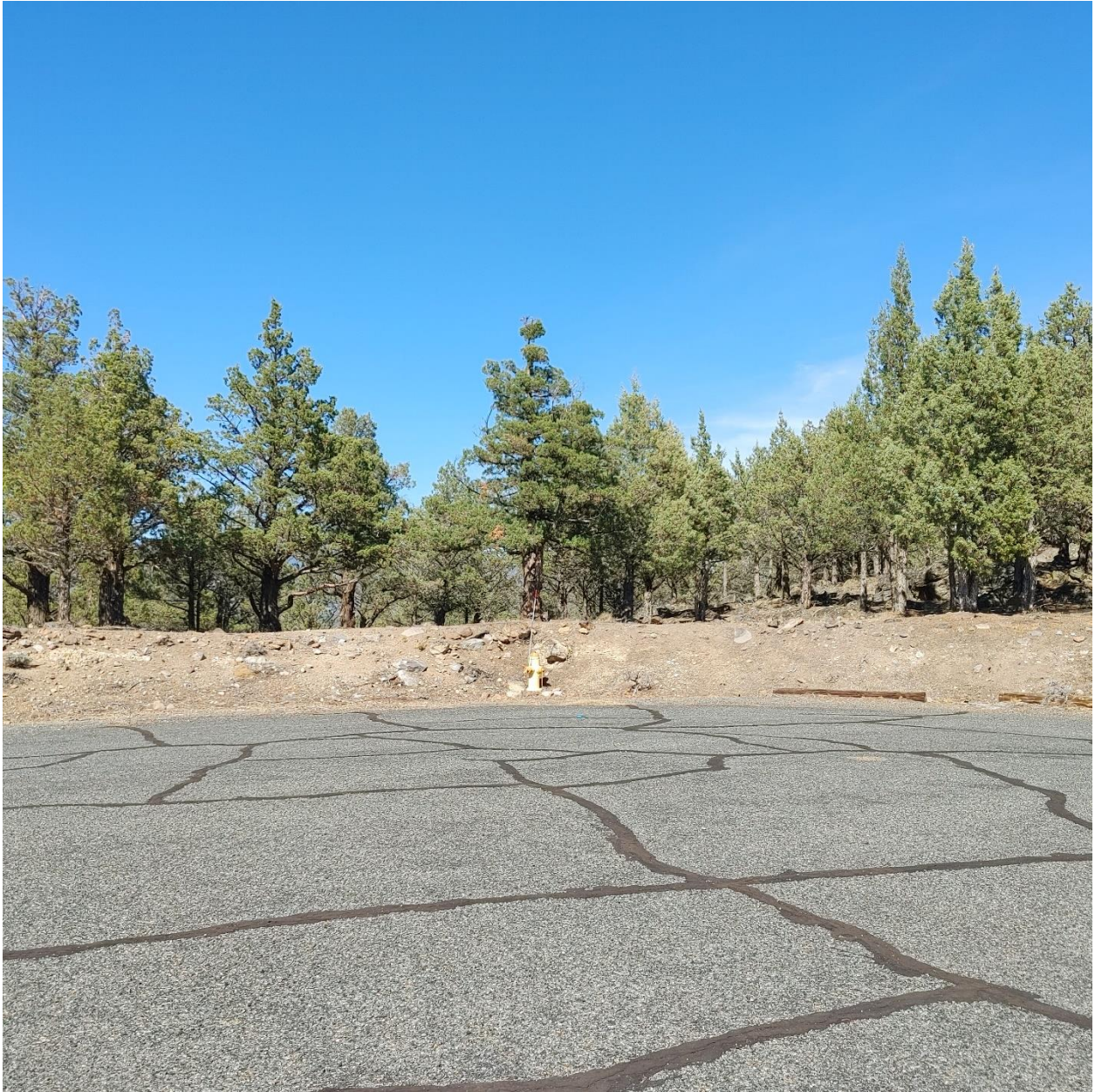
Photo 6: Looking North east from the cul-de-sac of Stone Crest Drive at fire hydrant #289 that will be replaced with a new fire hydrant. This fire hydrant is surrounded by asphalt, small rocks, gravelly soil, and juniper trees. The soil directly around the fire hydrant will be disturbed as all parts of the hydrant will be replaced down to the elbow in the ground.
